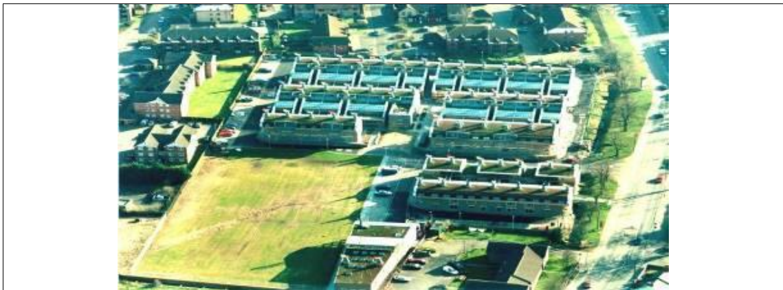
Figure 5.6: An arial view of Pool Houses (Bed ZED), showing the residential buildings, services and green areas.
