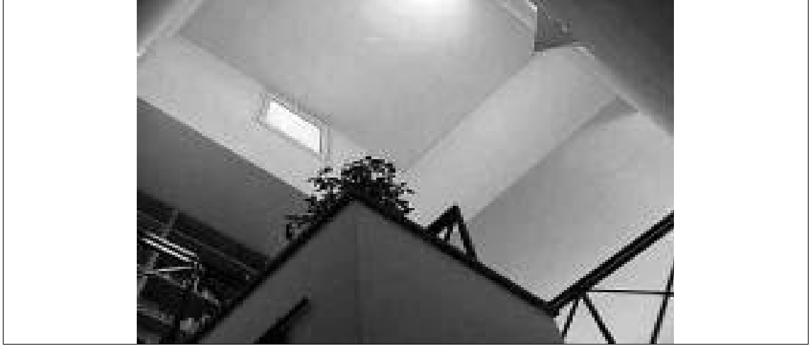
Figure 5.10: Windows on upper levels enable ventilation (cross, stack, and suction) during summer season nights
