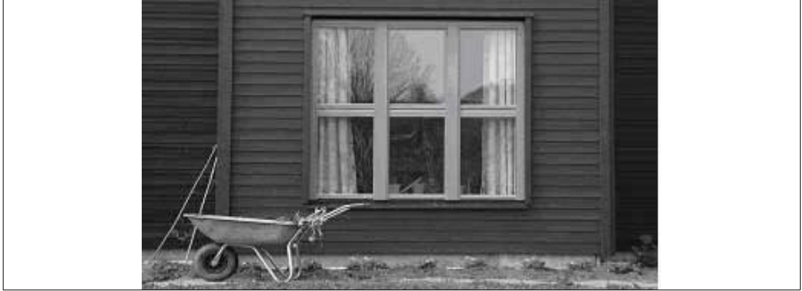
Figure 5.3: Windows at the end wall of Lindas Passive House Project
