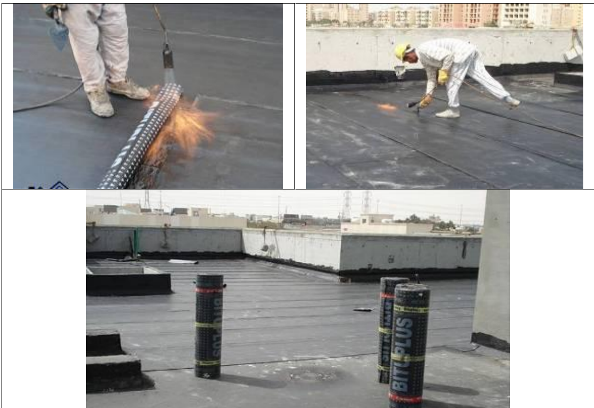
Figure 4.19: The process of fixing waterproof rolls over the foam concrete
