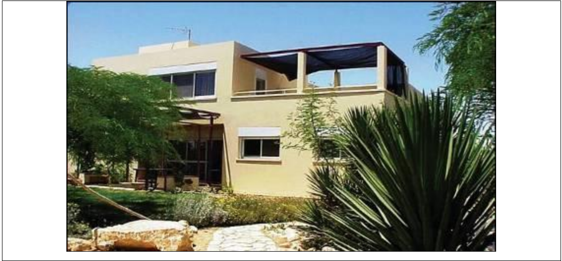
Figure 5.5: General view of Meir House, Negev Desert
