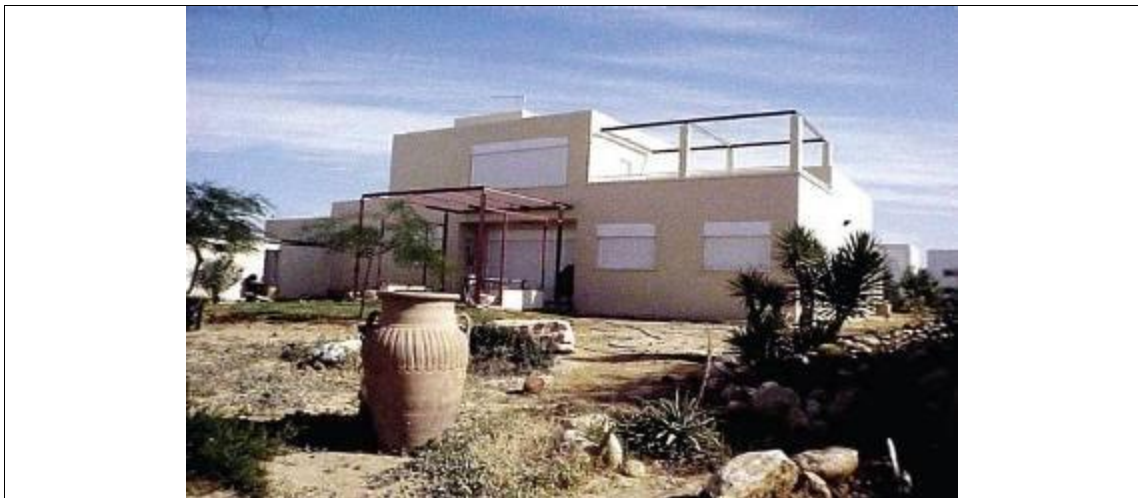
Figure 5.9: The shutters lowered in Meir House Source: (Roaf, 2007)
