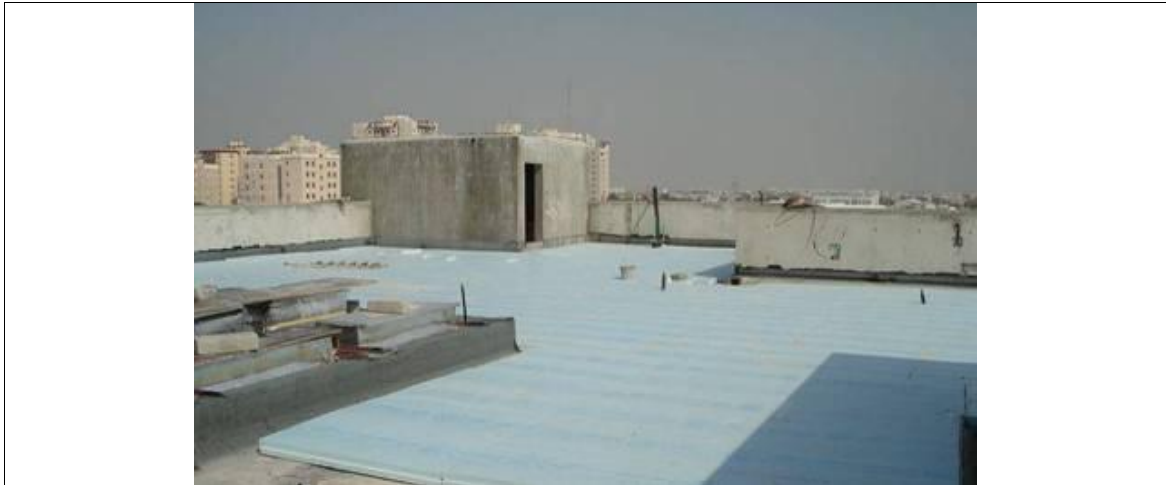
Figure 4.17: The process of installing insulation boards over the roof
